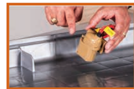
Limit Switch Installation
